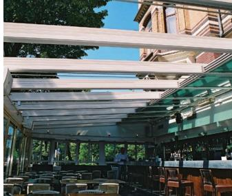
The beams are made of fiberglass, which has a 400 times better Insulation factor then aluminum. They can stretch over 20 feet and by using a support beam it can stretch much further. The 4 panel beam has a height of 215 mm and a width of 100 mm.
